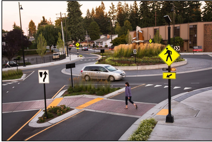
Figure 8. Example of a roundabout with mountable center curb and lighted crosswalks.
