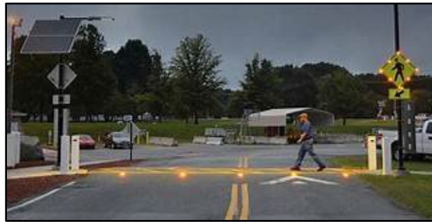
Figure 5. An example of a lighted crosswalk
