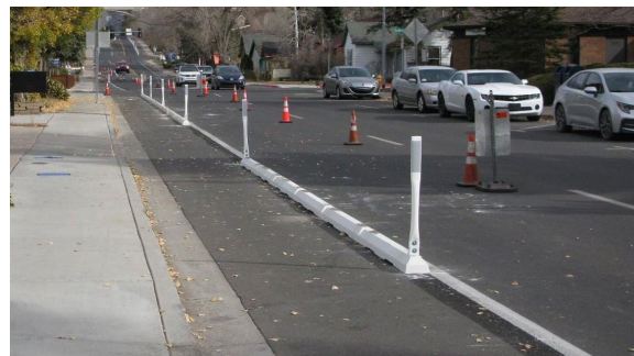
Figure 6. Example of a curb protected bicycle lane with driveway gaps on Butler Ave in Flagstaff.
